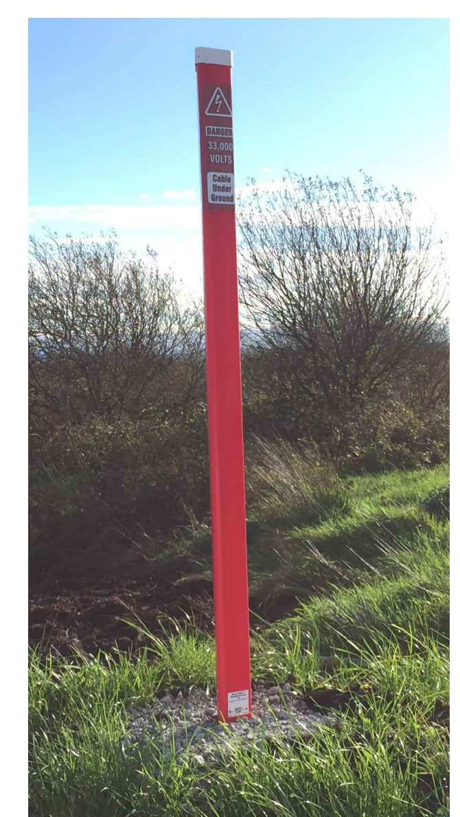
Typical Cable Marker Post
